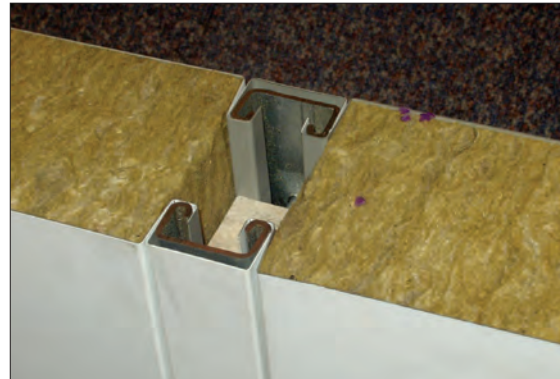
Figure 17: Insulated core panels – internal panel
