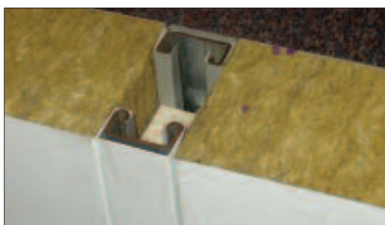
Figure 17: Insulated core panels – internal panel
