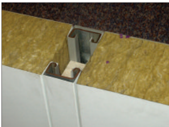
Figure 17: Insulated core panels – internal
