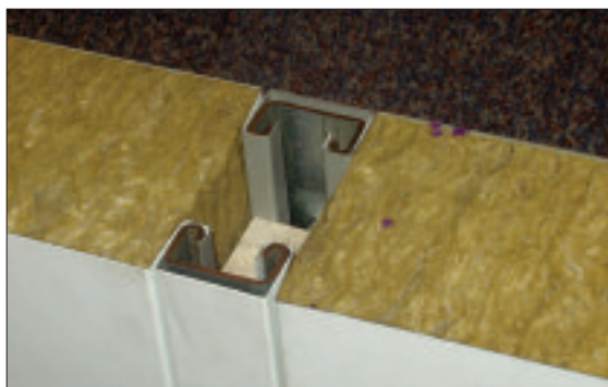
Figure 17: Insulated core panels – internal panel
