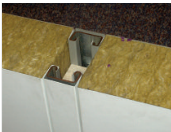
Figure 17: Insulated core panels – internal panel
